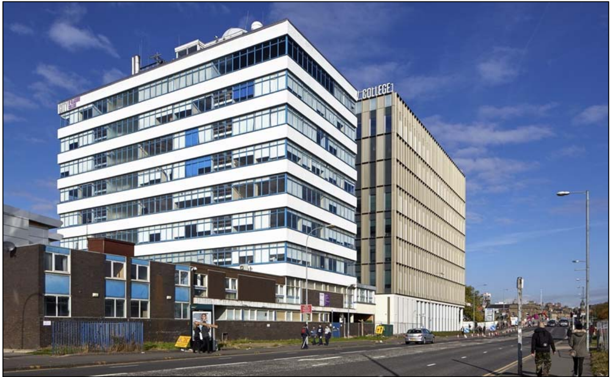
Figure 23 – Old College building before demolition
