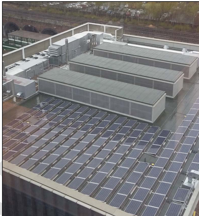
Figure 7 – PV panels located on workshop roof
