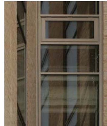
Opening light glazed into curtain walling
