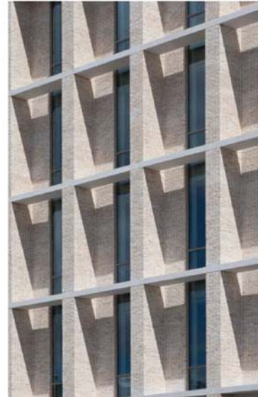
Precast cills and brise soleil
