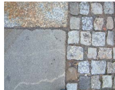
Granite pavers and setts
