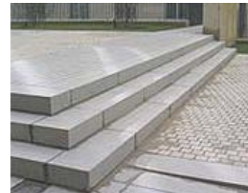
White precast concrete steps, granite pavers, setts & stainless steel handrails
