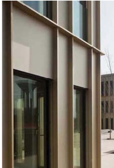
Insulated metal cladding and expressed fins
